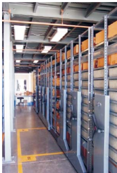
Economical, open-style drive column's give clear visibility into the items being stored on Mt. Home AFB's Mobile Aisle System.
